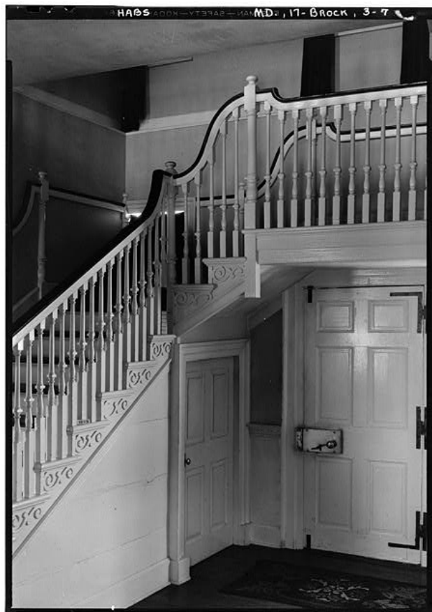
Staircase at Harmony Hall, 1934 Historic American Buildings Survey
