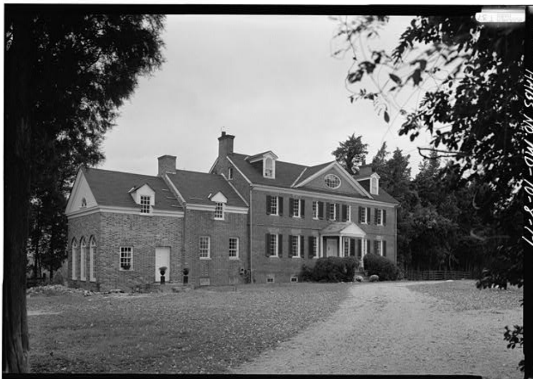
Harmony Hall with Collins Additions, 1934 Historic American Buildings Survey
